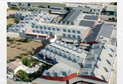
Roof system with 120 DEGERtracker 8.5, Spain
